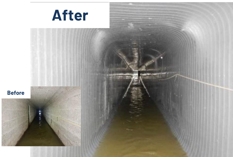
Renewal of old sewer pipes from the inside
